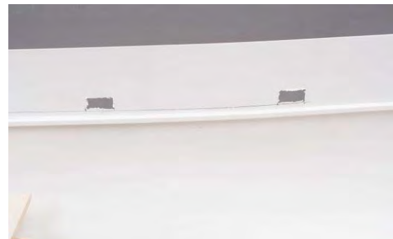
Fig. scuppers cut out, from inside
